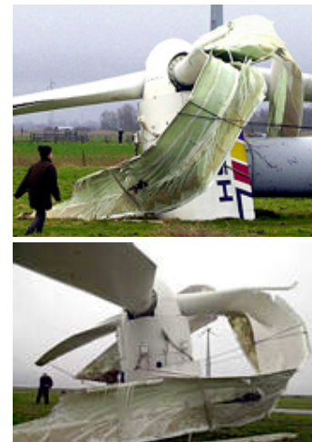
WKA turbines in Eifel, Germany, after Jan. 28, 2002, windstorm.
