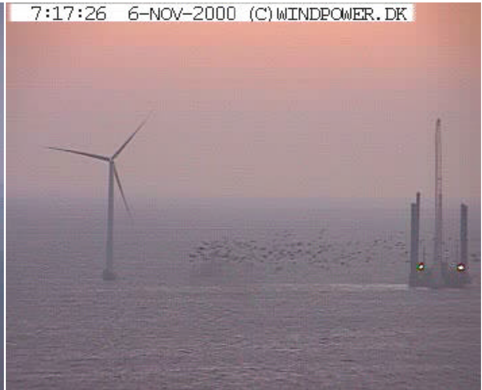
One turbine completed
